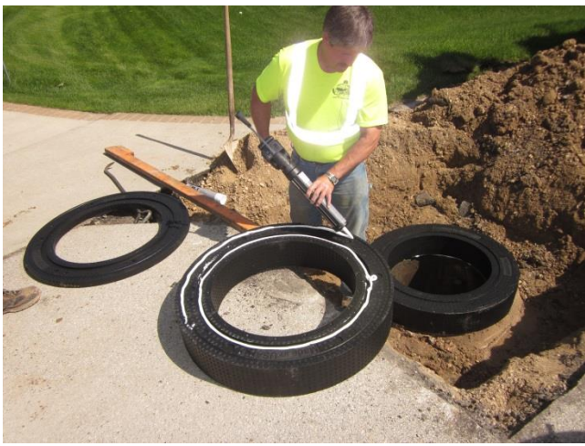
7. Apply a ¼" to ½" bead of M-1 adhesive to the groove and to the outer glue trench of the next Grade Ring or proceed to step 8 for Finish Ring
