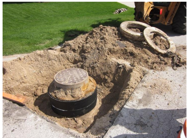
12. Install and center the manhole frame casting. With installation complete, backfilling and paving may proceed immediately.
