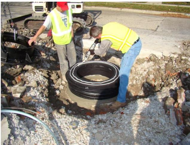
**11. Place two ½" beads of M-1 adhesive on the top surface of the Finish or Angle Ring prior to setting the manhole frame casting.**
