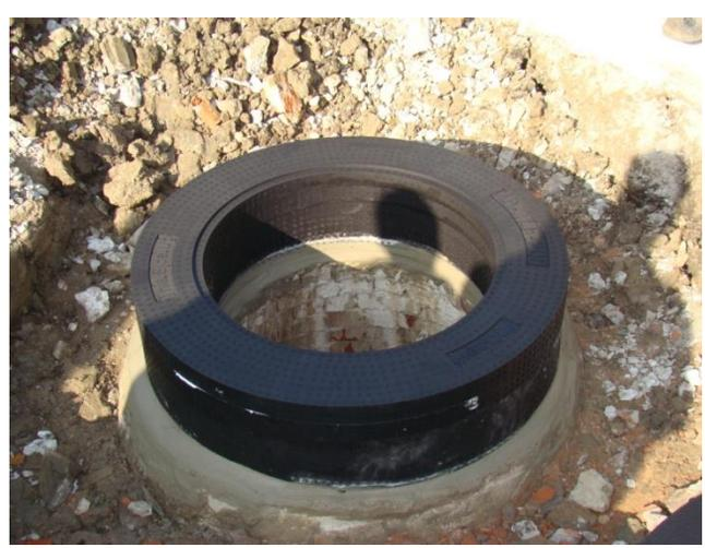
**8. Apply M-1 as before to the tongue and outer glue trench. Position the Finish Ring with the grooves down onto the Grade Ring.**
