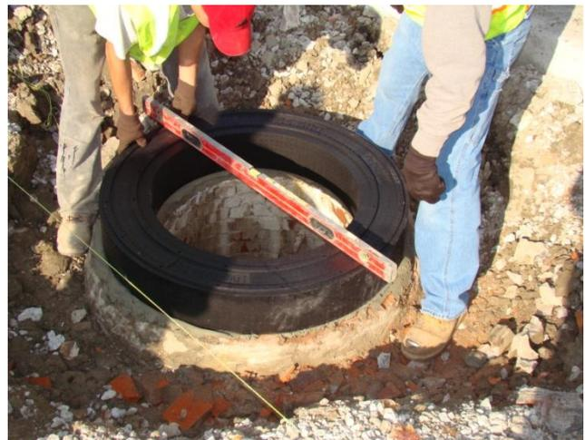
4. Position the first Grade Ring by embedding it directly into the mortar. Center the ring and make sure that it is level.
