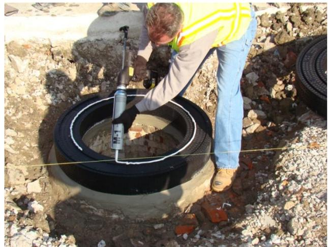
6. Apply a 1/4" to 1/2" bead of M-1 adhesive to the tongue and a to the outer glue trench of the next ring. Install the Grade Ring grooves down.
