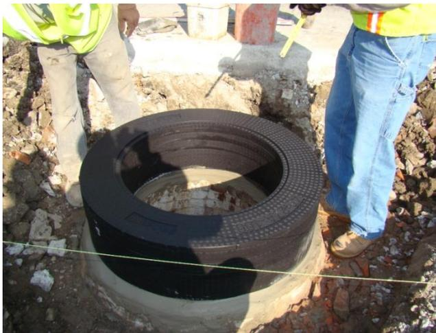
5. Dry stack the selected rings and verify the measurements to ensure the desired elevation has been attained. Apply paint alignment mark.
