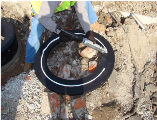
**9. For Angle Rings, place a ¼" bead of M-1 into the groove on the underside of the Angle Ring and to the inside shoulder of the Finish Ring.**
