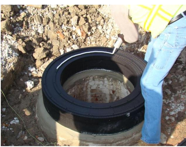
**7. If multiple Grade Rings are required, repeat step 6 until all Grade Rings have been properly installed and then proceed to step 8.**
