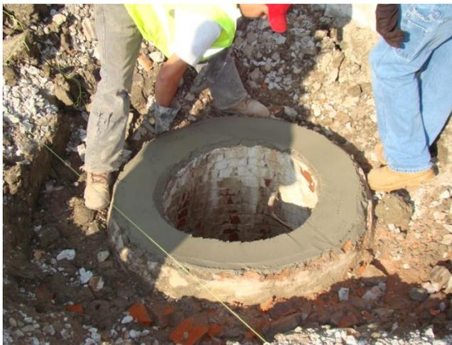
3. If the brick surface on top of the manhole is irregular, place a 1/2" thick bed of non-shrink mortar or grout on the surface and rough in.
